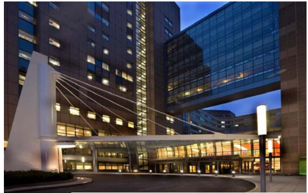
Photo courtesy of Turner Construction
